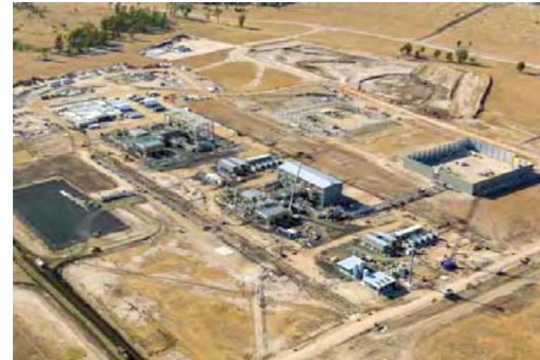
Condabri South - Gas Processing Facility
