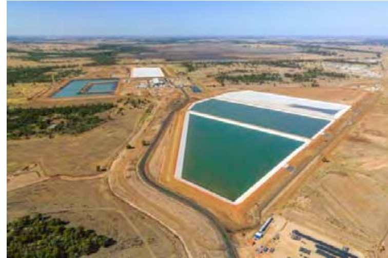
Condabri Central - water and brine ponds
