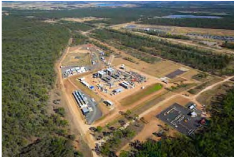
Talinga – Pipeline Compression Facility, Gas Processing Facility in background
