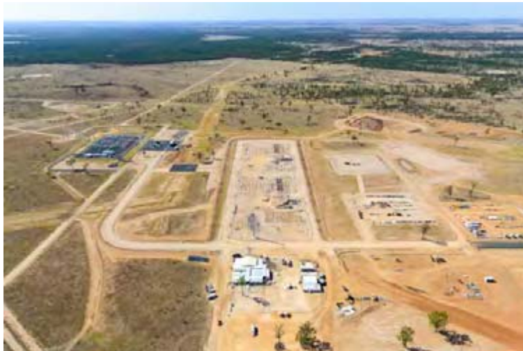
Condabri North - Gas Processing Facility
