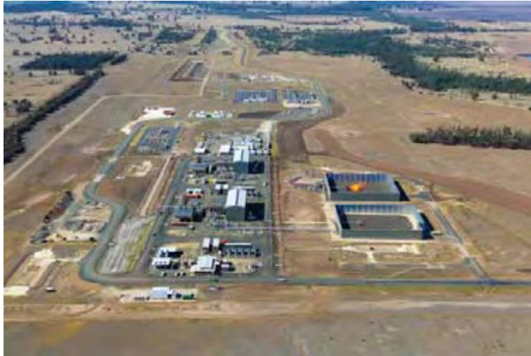
Condabri Central - Gas Processing Facility
