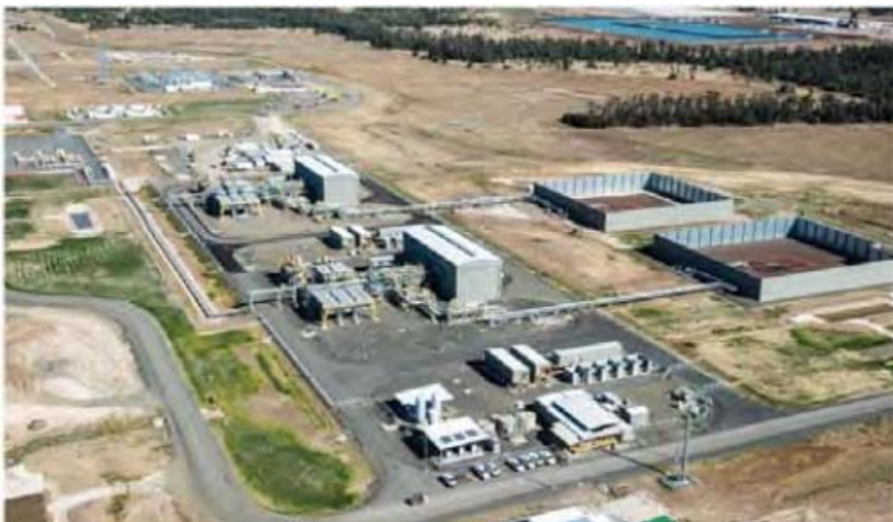
Condabri Central Gas Processing Facility
