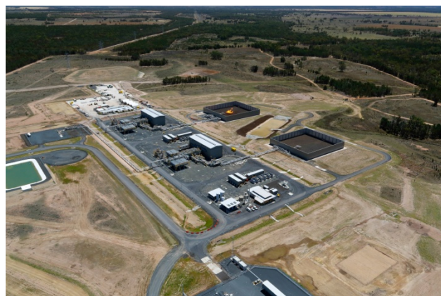
Orana Gas Processing Facility
