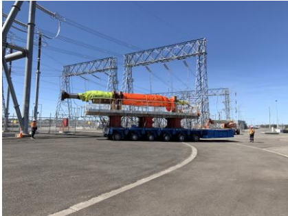
Old rotor being removed at Mortlake
