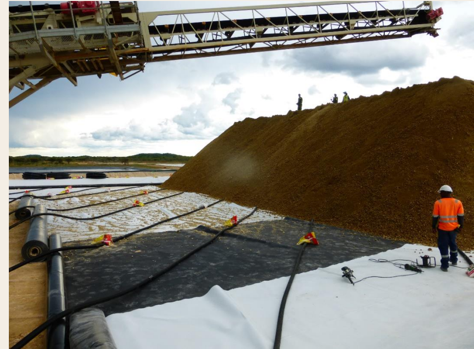
Figure: Example of Heap Leach construction
