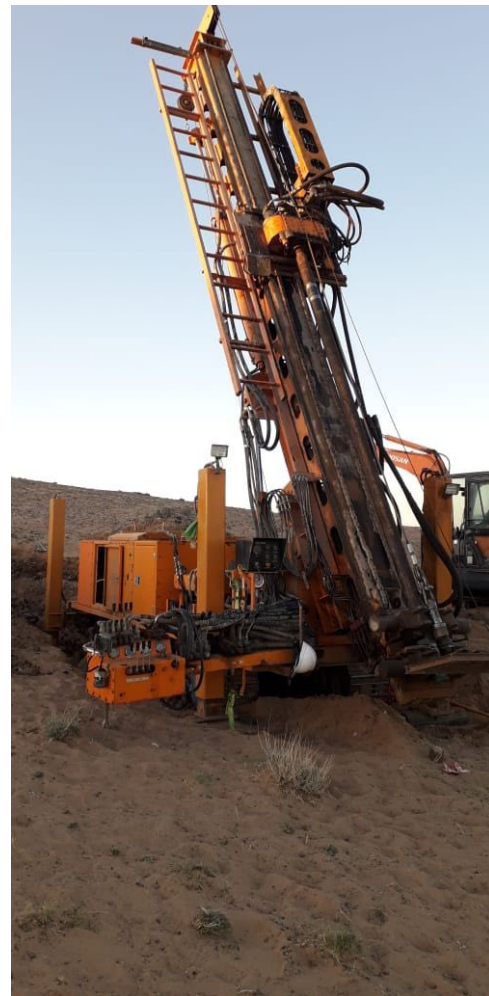
Image 3. Drilling rig Setting up over the first hole
