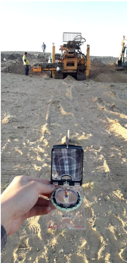
Image 2. Preparing first drill pad
