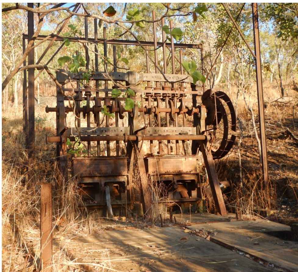
Plate 3 – 1904 Stamp Battery that was part of the Spring Hill Mining Centre processing hub
