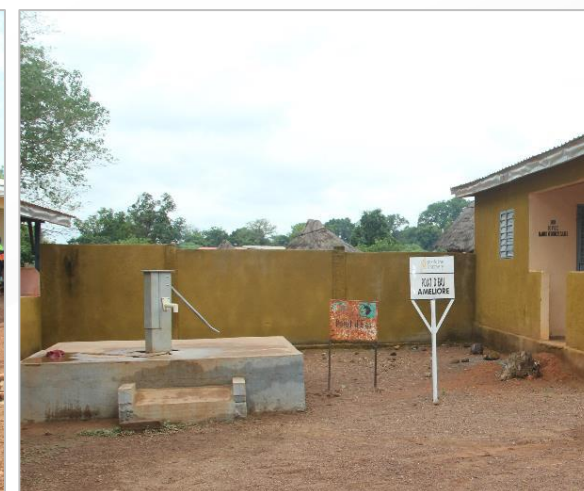
Installation of additional water bores
