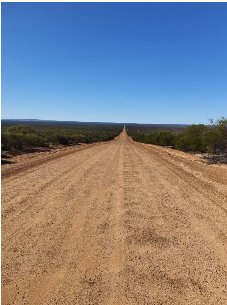
Mt Adams Road which intersects the Beharra Tenement
