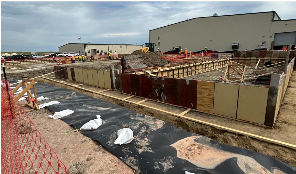
Figure 2: Crews installing forms in preparation for upcoming concrete pours at Ross CPP site
