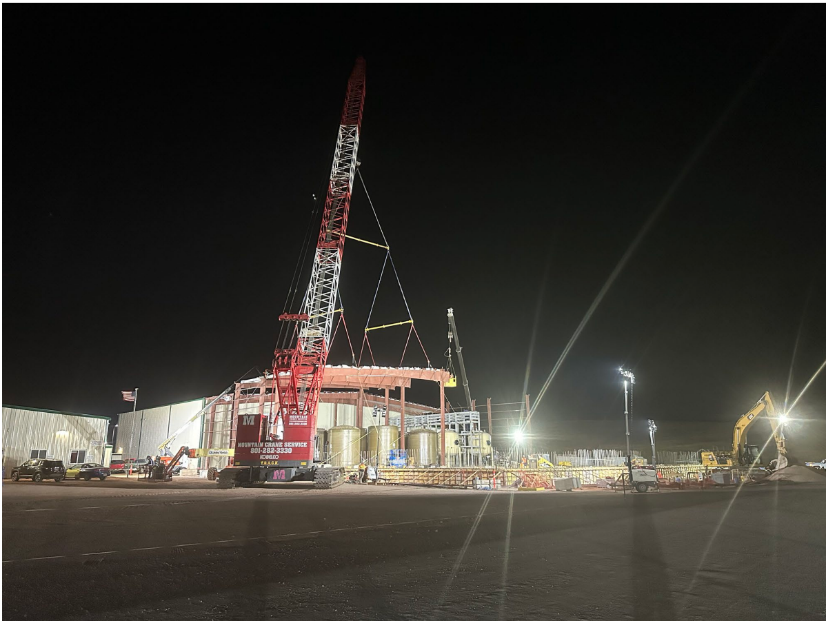
Figure 1: Nighttime placement of roofing structure
