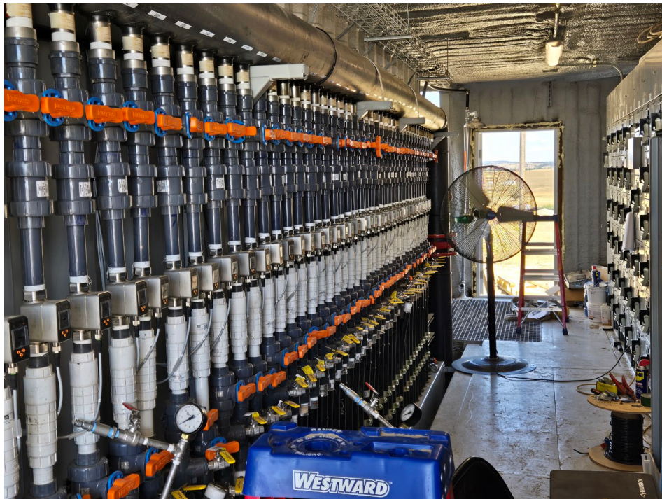
Figure 5: HH-11 interior under construction in August 2024
