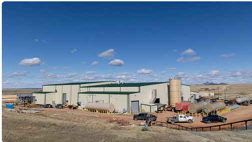
Central Processing Plant (Phase I & II)
