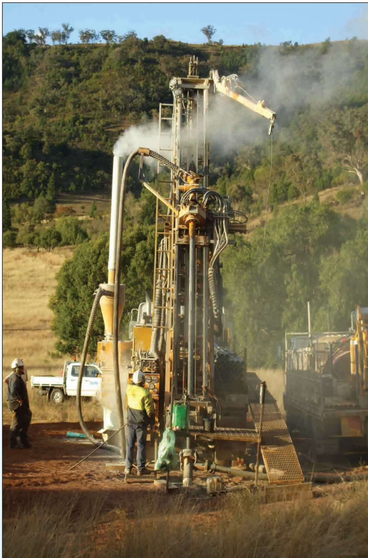
Figure 4 – Drilling at Kensington
