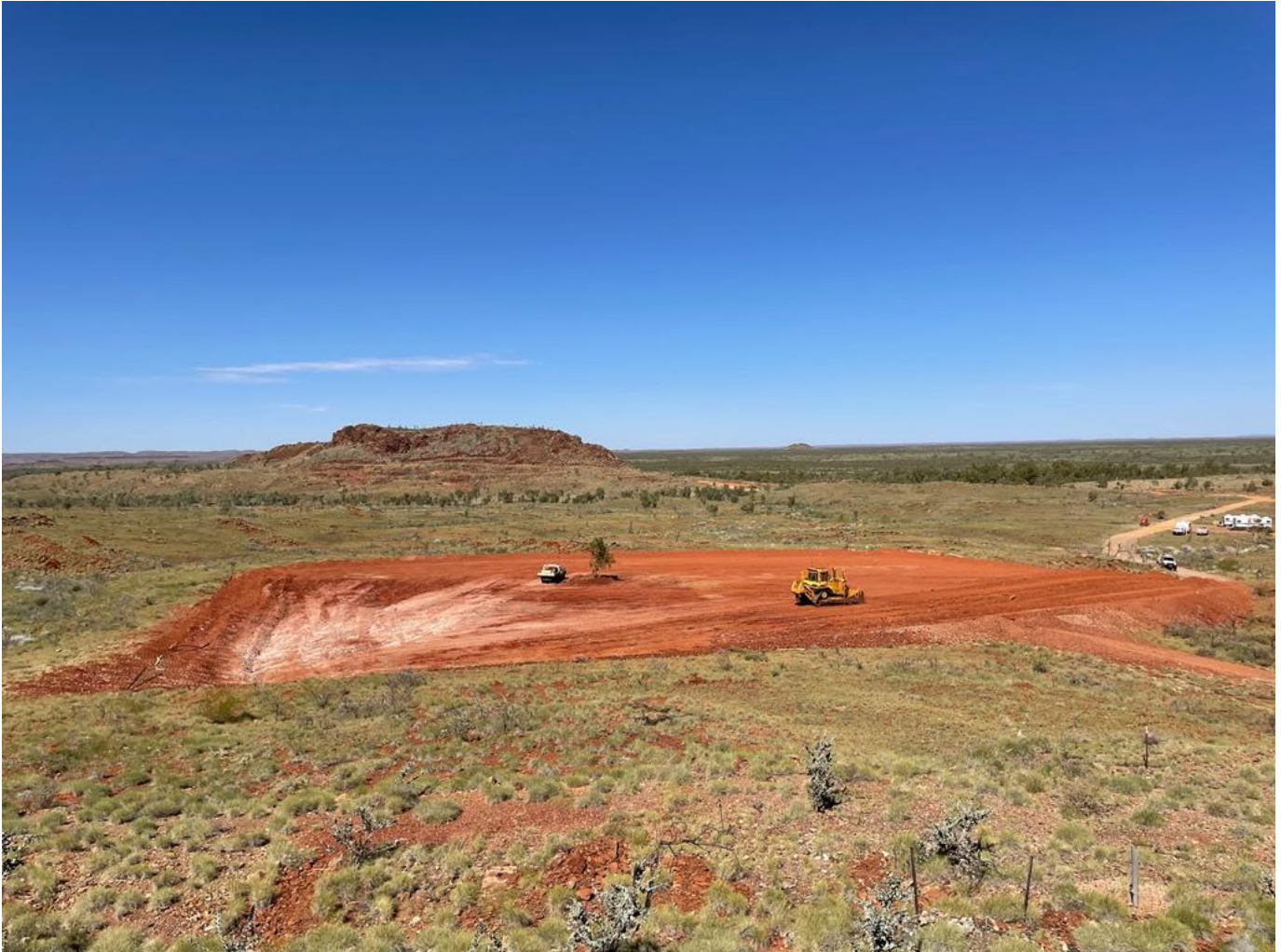
Figure 10. Exploration camp construction underway with levelling and compaction of 70m x 70m area in preparation for dome-sheltered core yard, accommodation, ablution block, workshop and offices. The prominent hill in the background is the part of the Main Hill prospect. View looking south.
