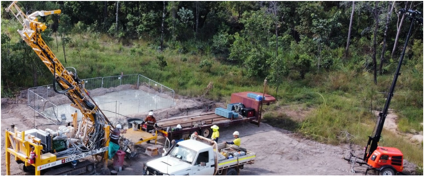
Figure 2: Southern Target 2023 drilling (UDR650 rig)
