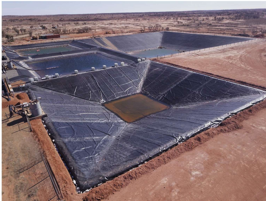
Photo 1: Completed relining of PLS pond at White Dam Gold Project, South Australia.
