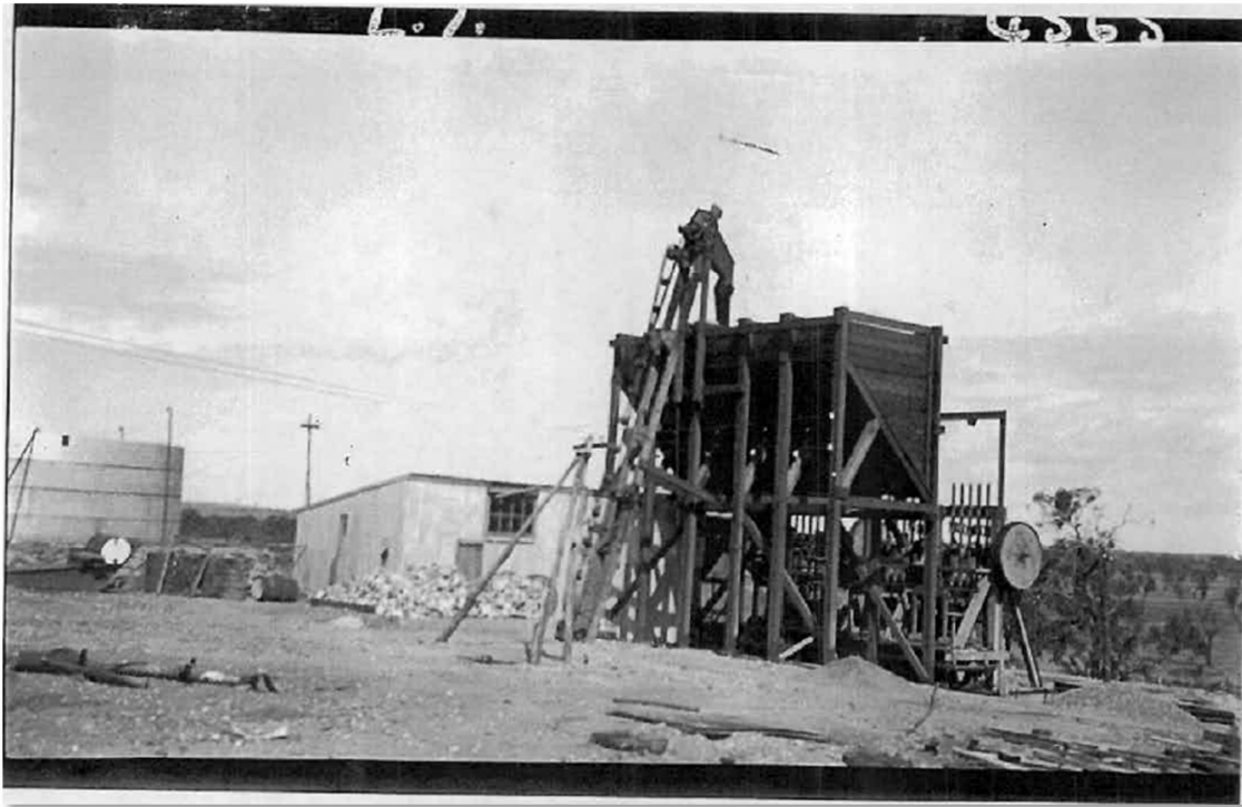
Figure 3: Power House, Ore Bins and Twenty Head Battery circa 1934
