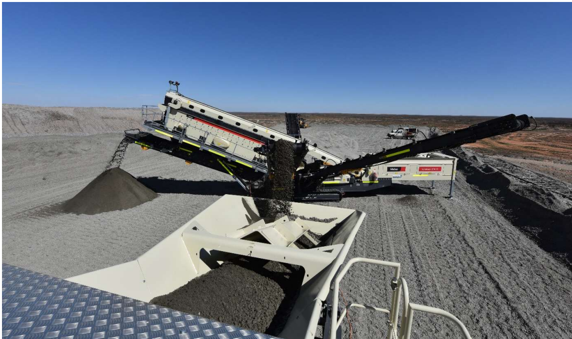
Figure 1: Screen and cone crusher being commissioned at Heap Leach pad
