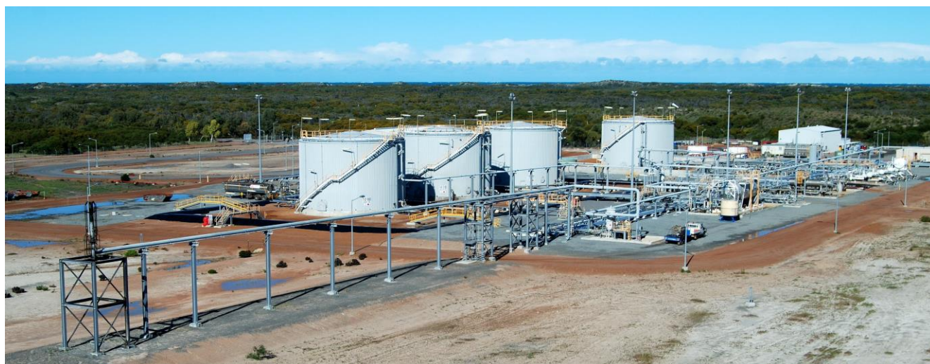
Figure 1: Arrowsmith Stabilisation Plant. Note the two outer tanks will be refurbished
