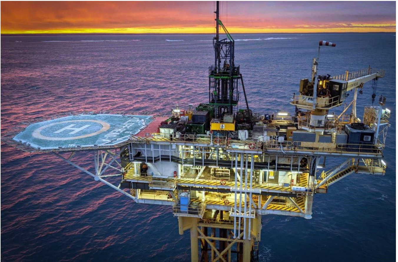
Figure 1: Cliff Head Alpha with HWU installed
