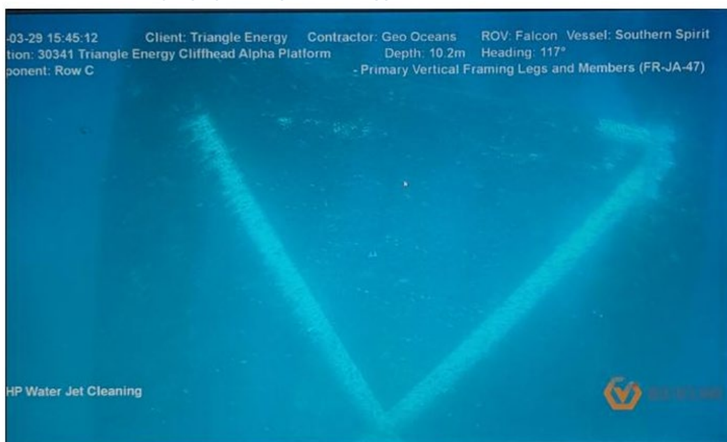
Photo 2: Underwater photo of structure after marine growth cleaning
