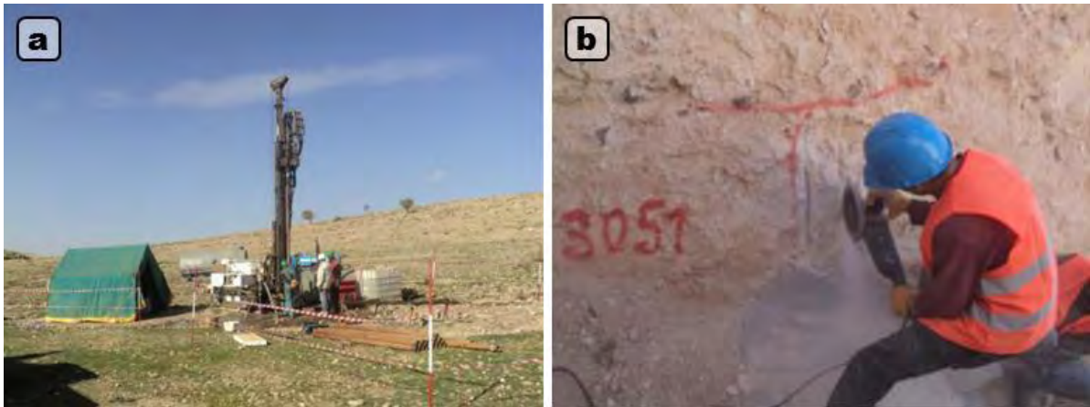
Figure 3-6: a) Drilling at Salsala, SADD-009; b) Chip-sampling in trenches, T006
