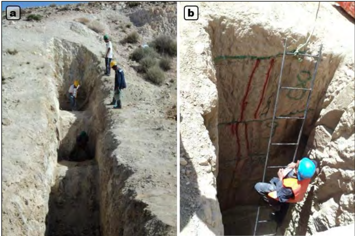
Figure 3-10: BEA (s.s.) Prospect, a) Trench T035 in Block A; b) Pitting in Block B
