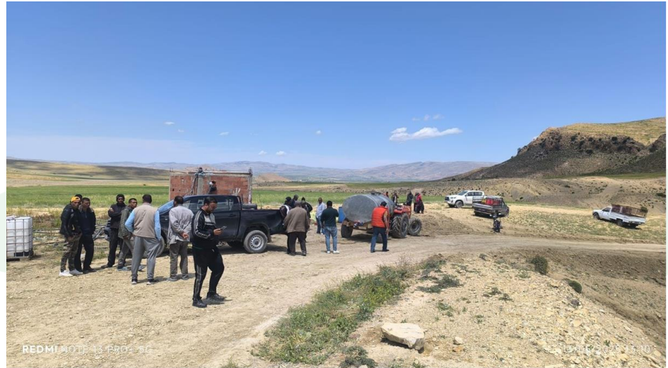
Repair of community water infrastructure by PhosCo
