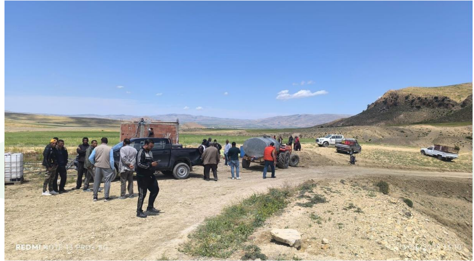
Repair of community water infrastructure by PhosCo
