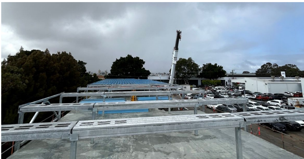
Figure 4: System Assembly at Forward St
