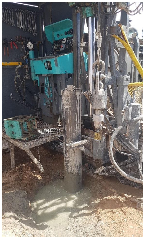
Figure 1. 8 inch diameter 30m steel pipe concreted into well hole.
