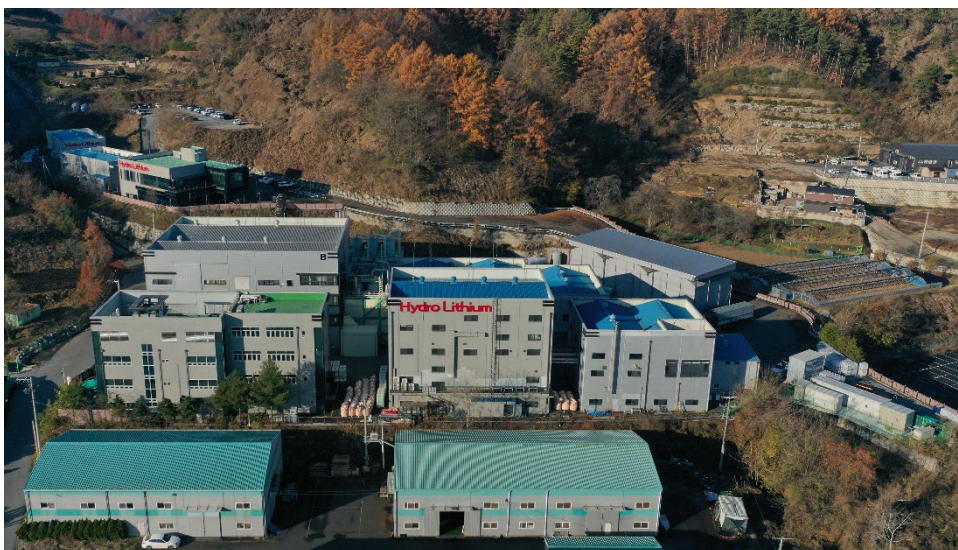
Figure 2: Hydro Lithium Refinery in Korea
