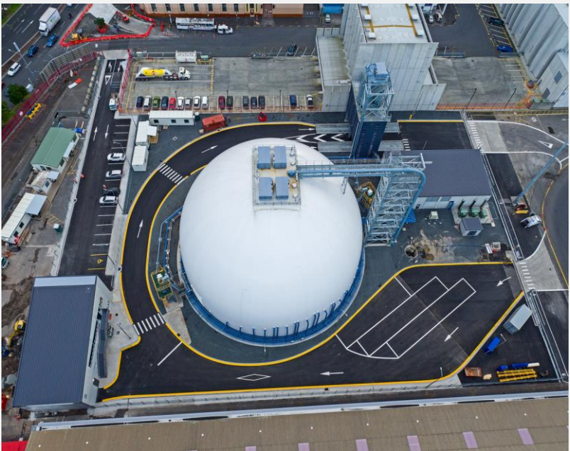
Holcim Bulk Cement Storage Facility (Auckland, New Zealand) with pneumatic loading/Unloading.
