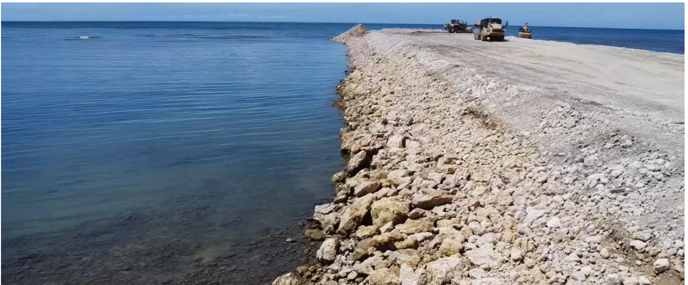
Pioneering Wharf at Central Lime Project
