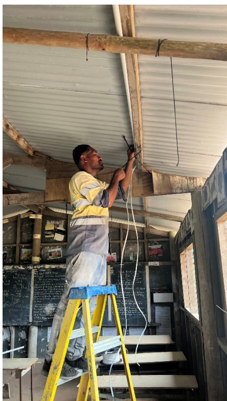
Electrician Completing Installation
