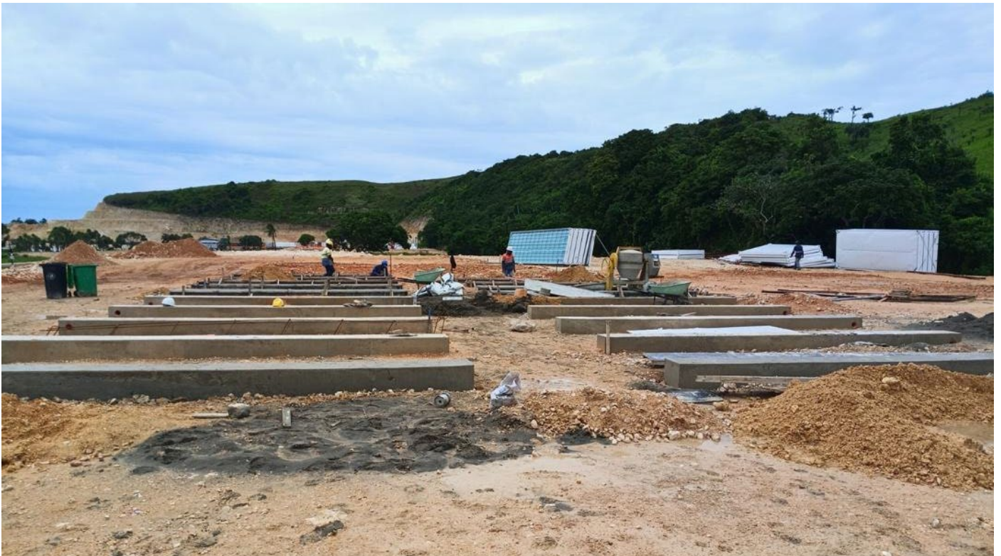
Image 2: Site foundations for the camp have been completed.
