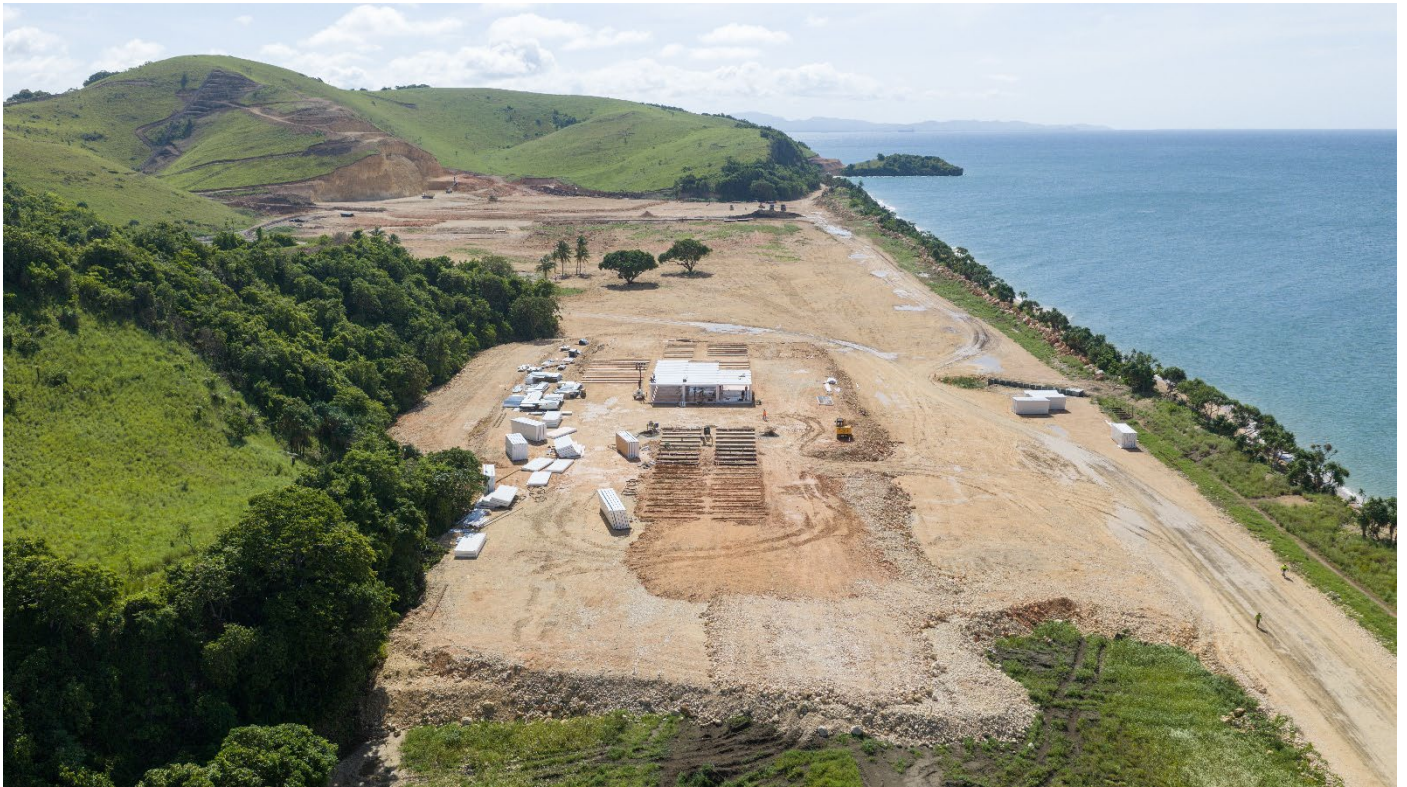
Image 3: Batch plant foundations and the construction and installation of camp prefabricated buildings.
