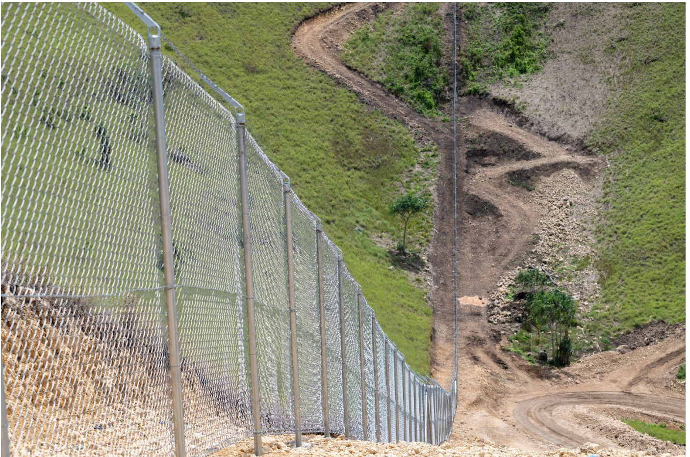
Image 4: Site boundary fence is nearing 50% complete.
