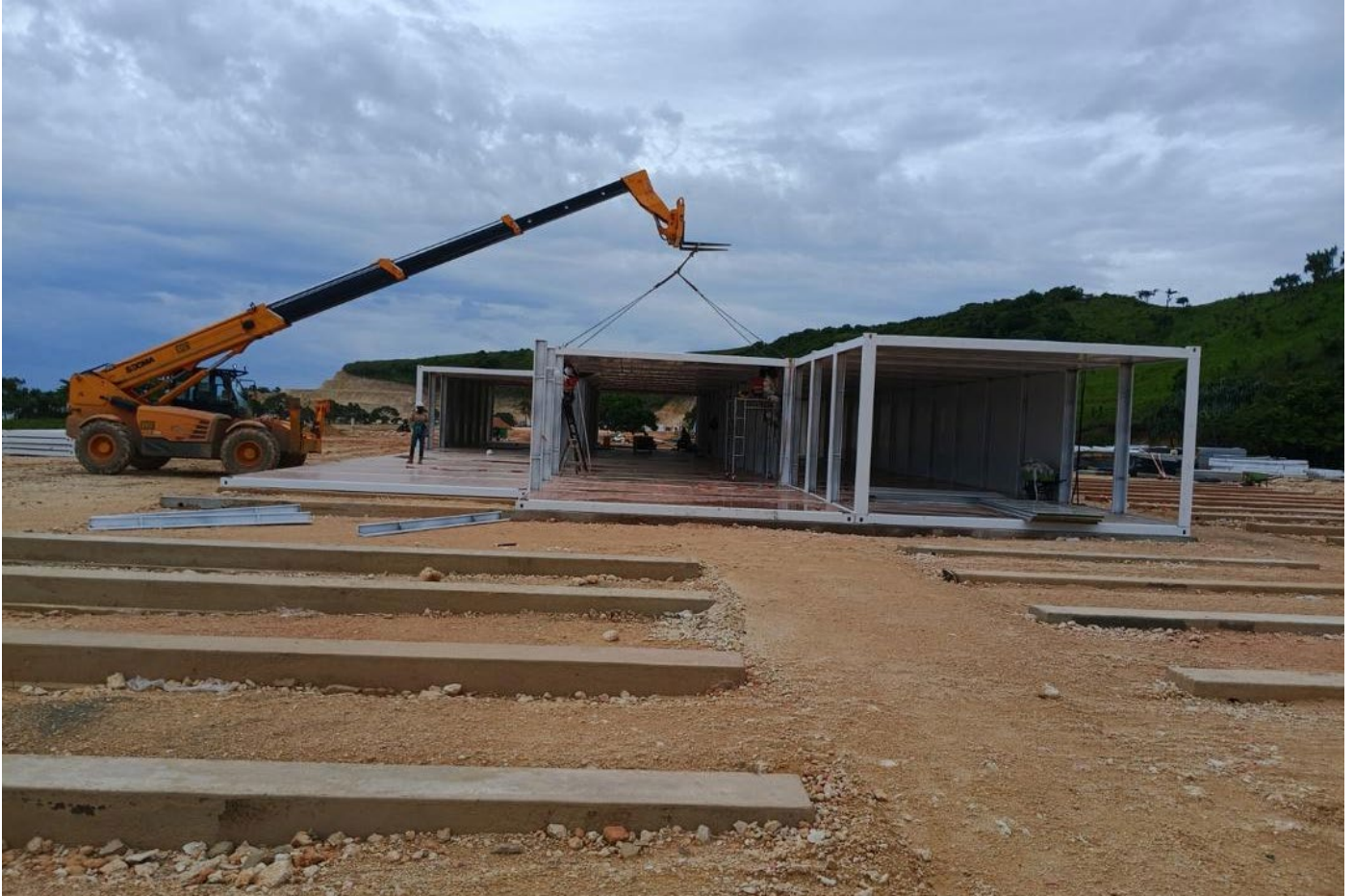
Image 9: Construction of the camp focusing on kitchen, ablutions, and office buildings.
