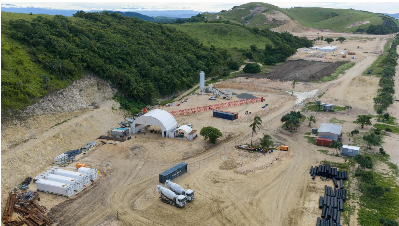
Photo: Construction progress at the Central Lime Project
