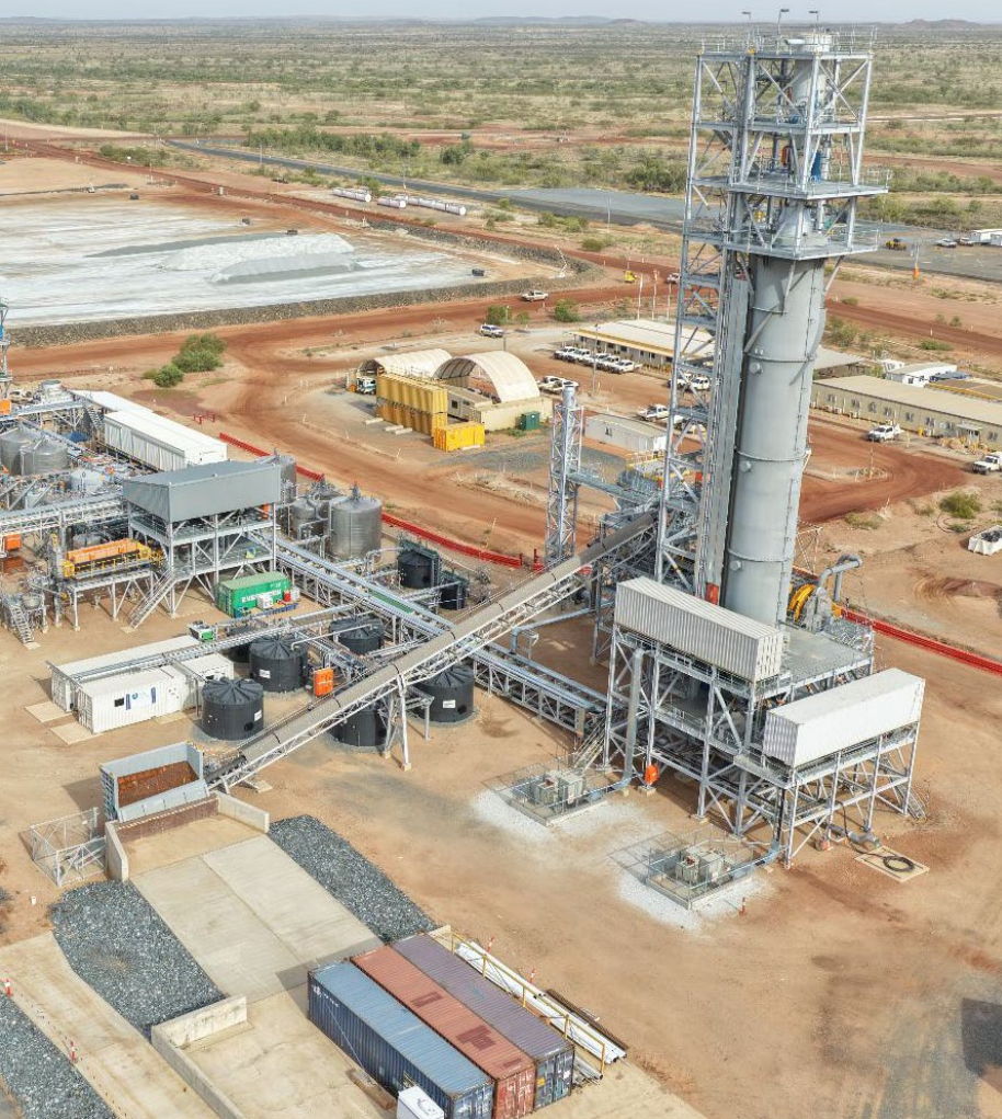
Image: Mid-Stream demonstration plant as at 29 January 2026
