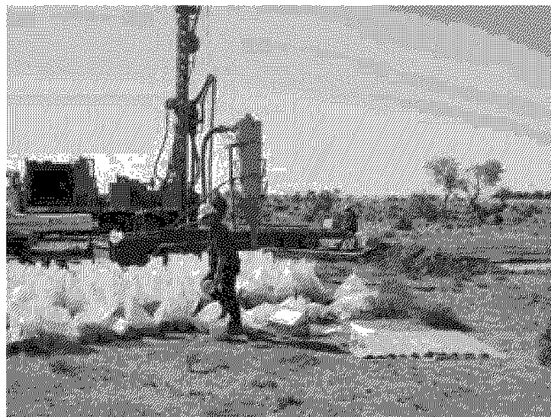
Drilling operations at Birthday Well Prospect
