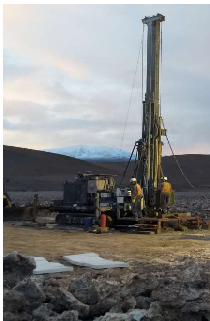
Photo 1 - Drilling Borehole PNN-VI-DW-02
