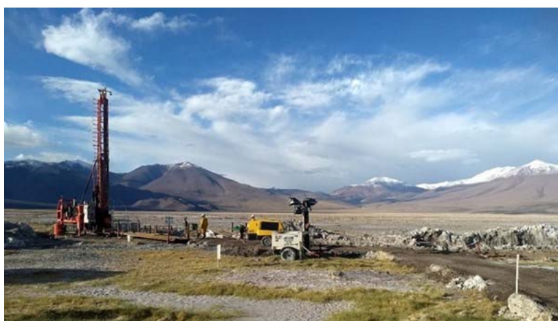
Photo 1 - Drilling Borehole PNN-SU-DW-01
