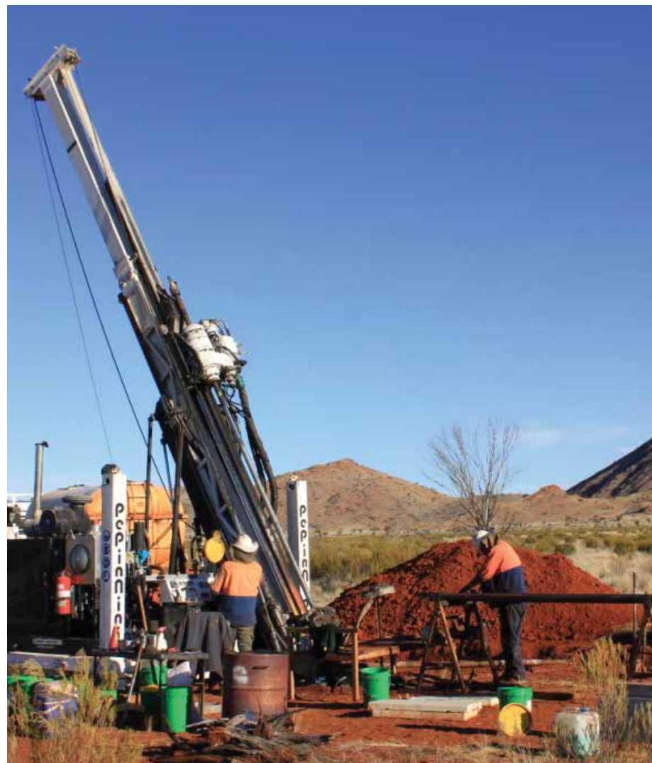
Photo 5 - PepinNini Diamond Core Drilling Rig
