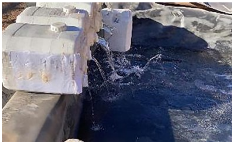
Photo 5 – 13 May - brine poured into prepared ponds with plastic liners
