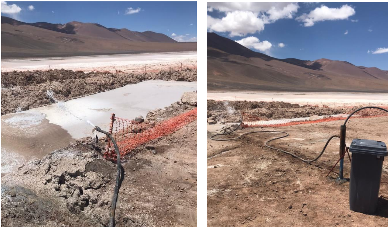
Figure 3: Airlift test of lithium brine flow rate, drillhole PM22-IN-002, Incahuasi salar
