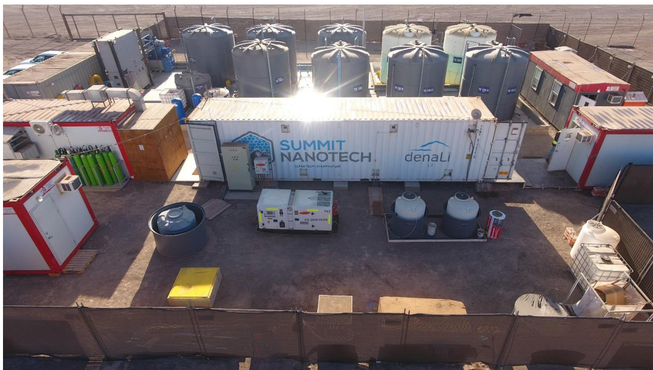
Figure 1: Summit Nanotech's DLE pilot plant facility in La Negra, Chile
