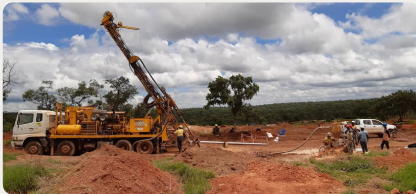
Alahiné Phase 2 drill collar AH21ARC126 (August 2021)
