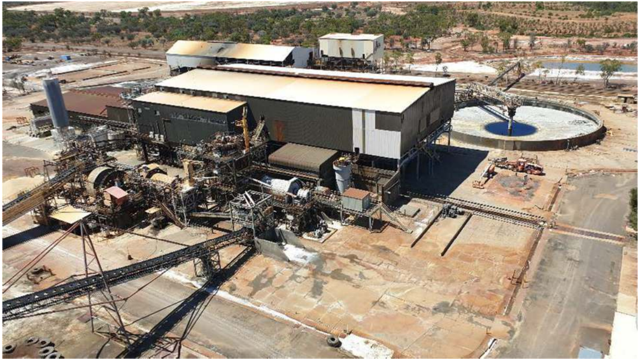
Photo 4 - Grinding, Flotation & Concentrate Areas
