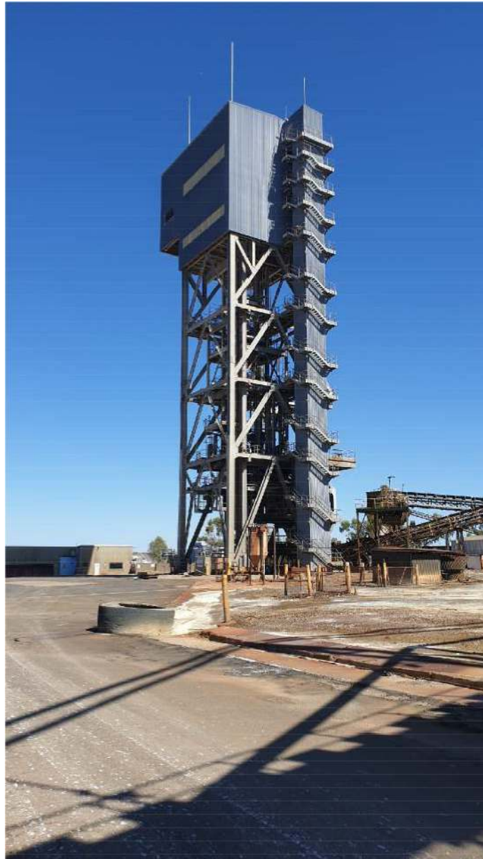
Photo 3 - Headframe & Surface Crusher
