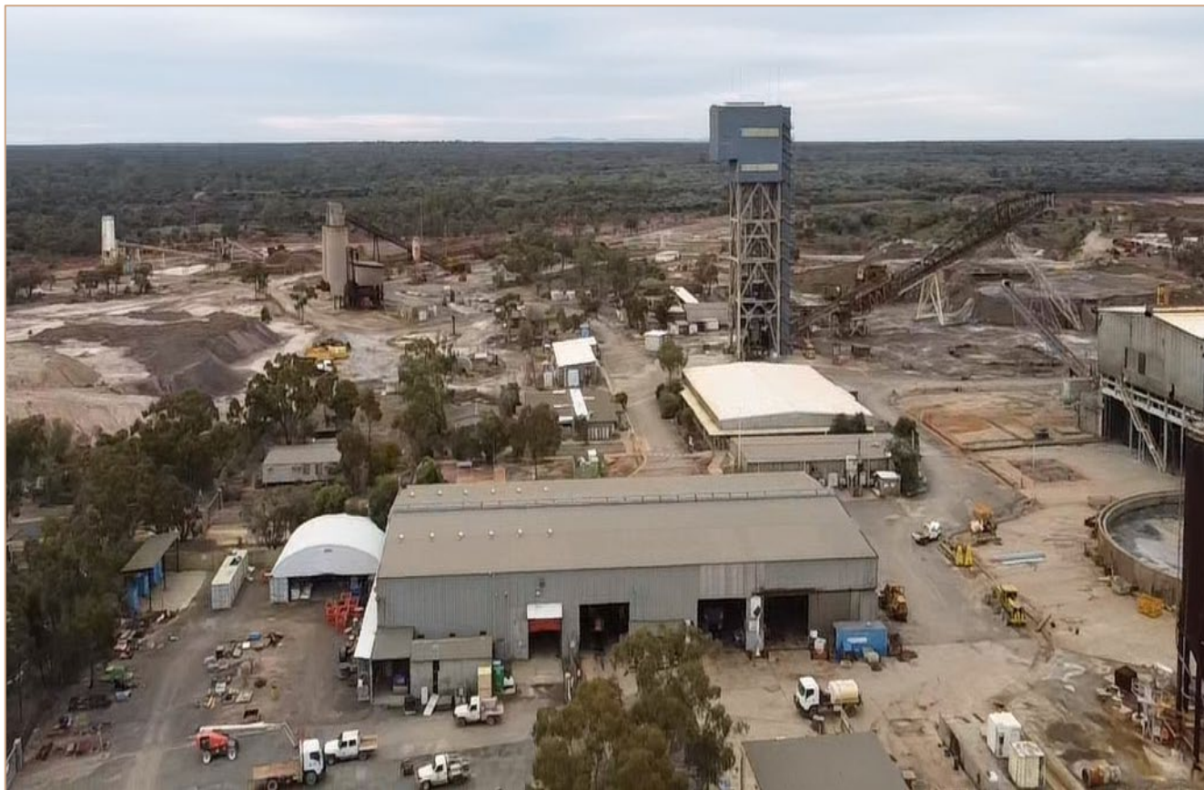
Figure 6: Endeavor surface workshop and headframe – November 2022
