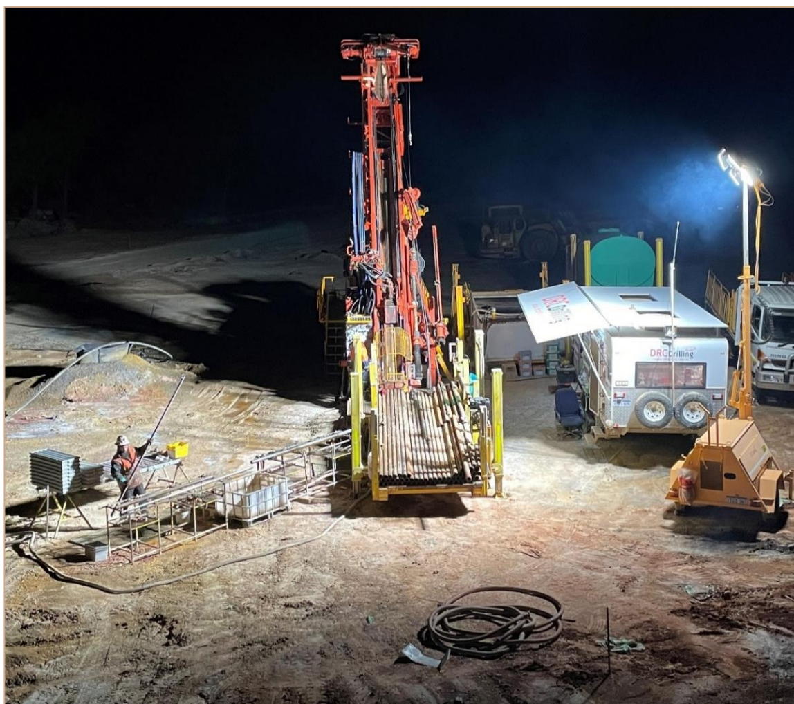
Figure 2: Upper North Lode - geotechnical drilling
