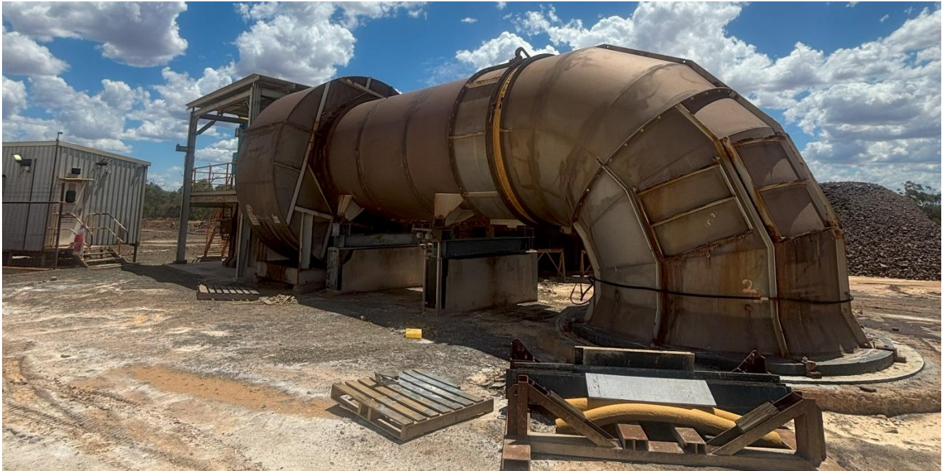
Figure 4: Refurbishment of vent fan No. 5 including sealing and replacement of foundations.
