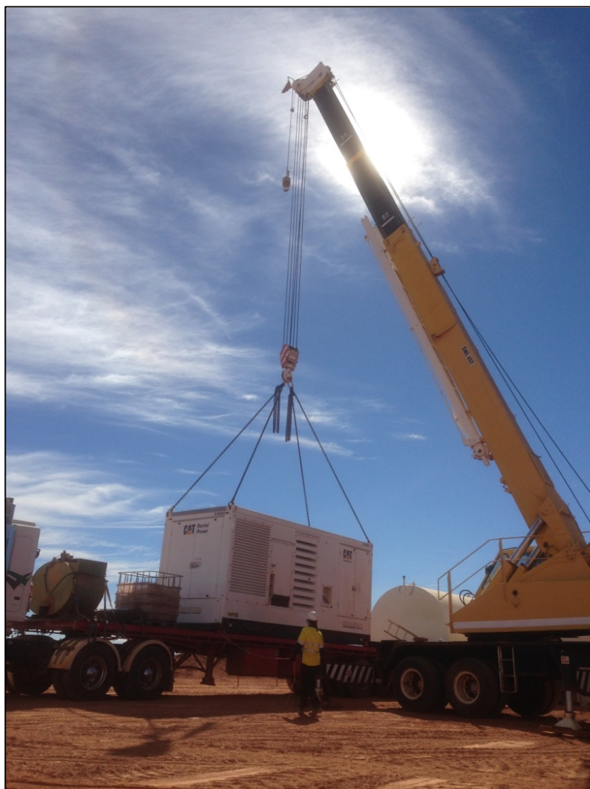
Figure 1. Generator Set being loaded into position with fuel tanks in the background to the right.
