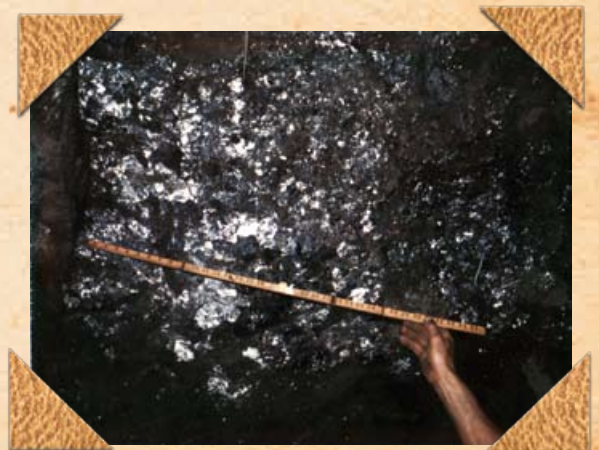
Measuring Galena ore body with yard ruler at historic Mary Springs Mine
