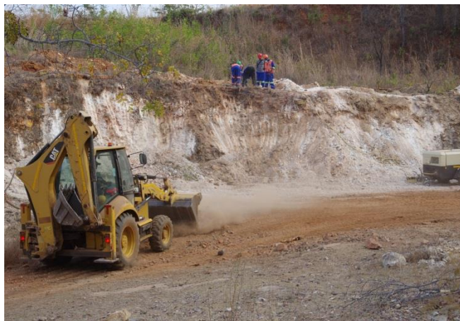
Preparing for the first blast
