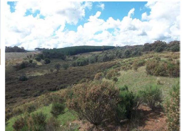
Tailings dam wall looking north
