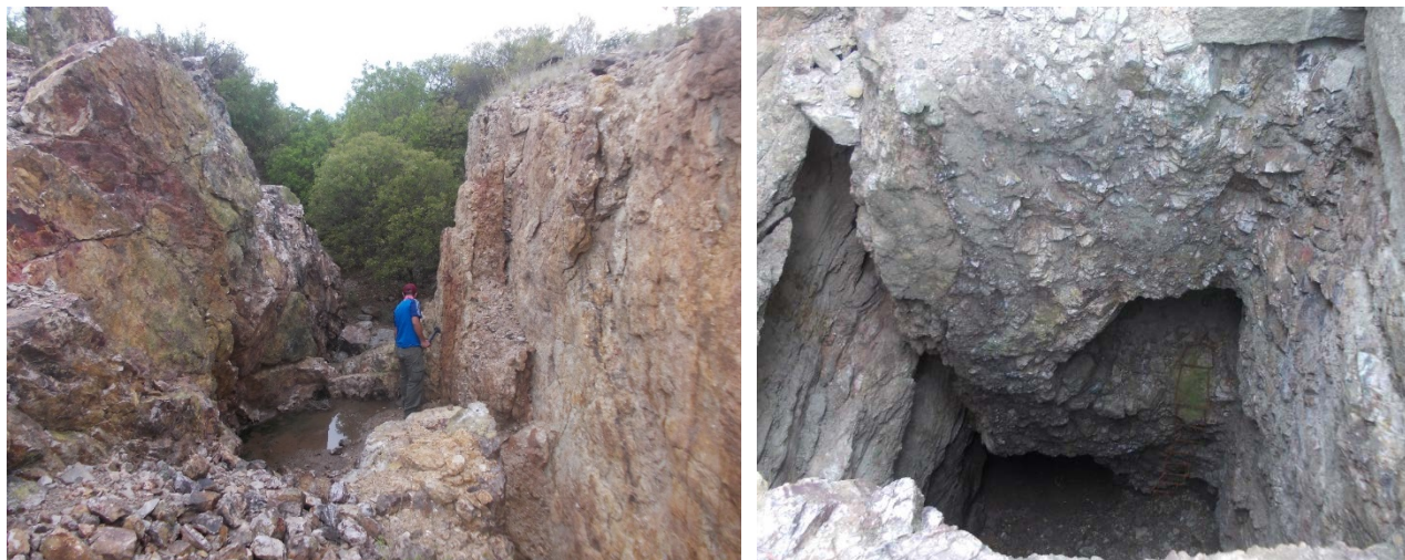
FIGURE 2B: NVM – SHAFT AND OPEN PIT
