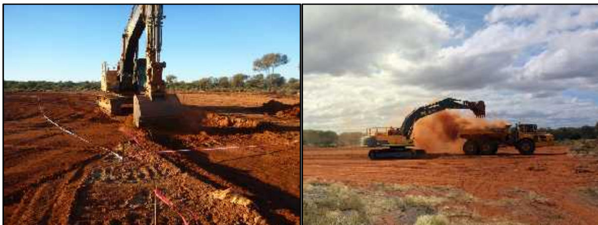
Figure 3 Mining Fleet commence construction of the laydown area and site works infrastructure facilities for the Lewis east open pit trial mining operation
