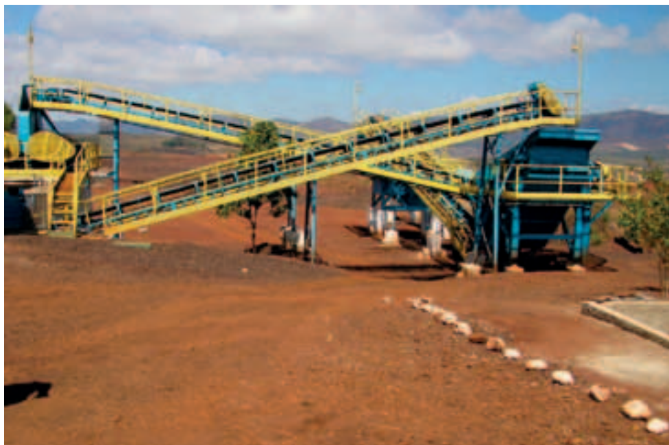
Figure 5.5_1 View across existing Ponto Verde plant
